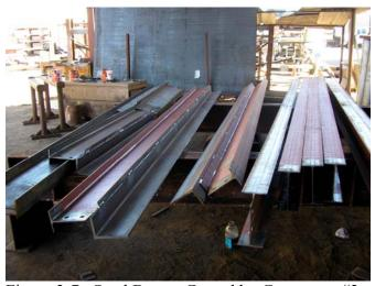
Figure 3-7. Steel Beams Coated by Contractor #2
